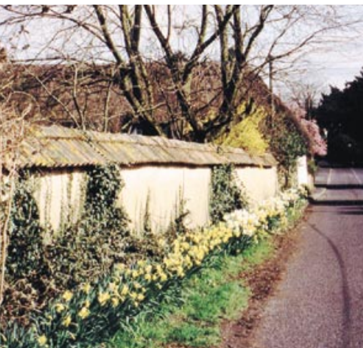
A typical tiled cob boundary wall.
