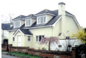
A modern house on Monxton Hill – the dormer windows enable the roof line to be as low as possible.
